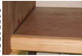
The picture to the right shows the use of a piece of machined softwood (50x50) along the front edge of a shelf which not only adds an attractive finish, but also provides added stiffening. This shelf is about 1.2m unsupported; for shorter lengths, smaller sized softwood can be used.
